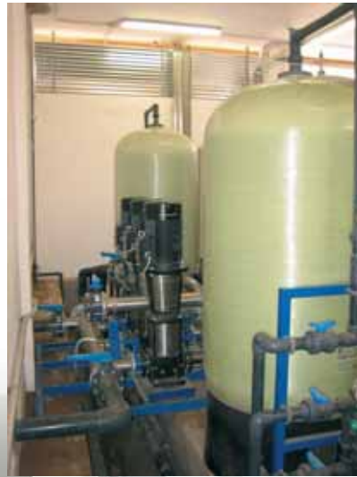
Above: Pretreatment line for sea water. Left: Remineralization and pressurization network. Below: Group of reverse osmosis lines
