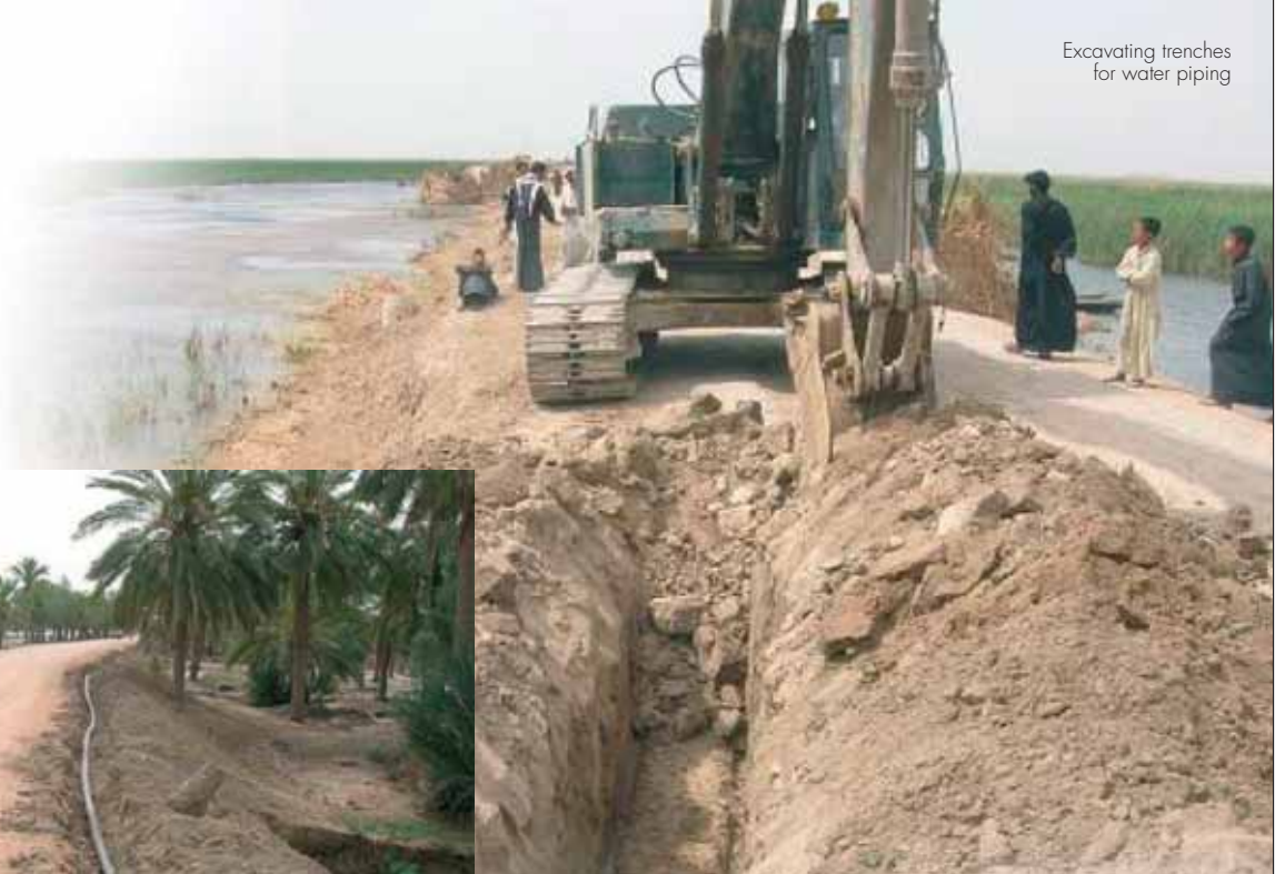
Piping being layed HDPE
