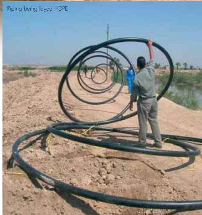
Water distribution piping being layed
