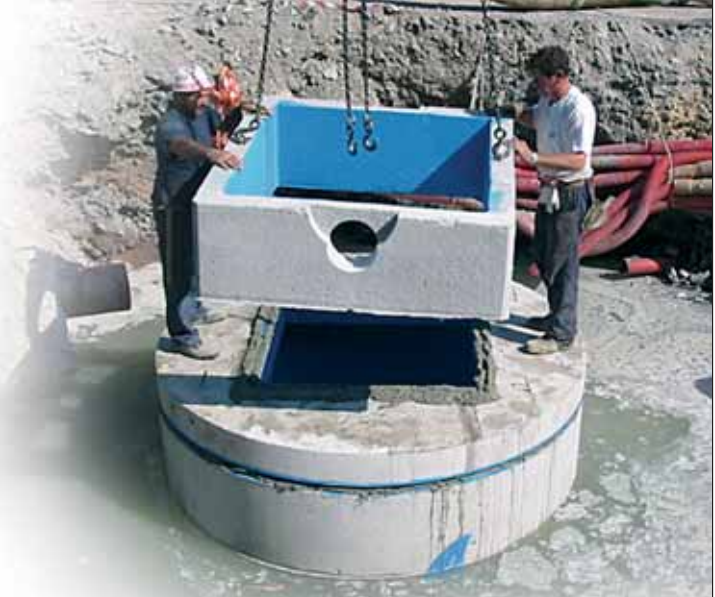
Installation of a lifting station in groundwater.
