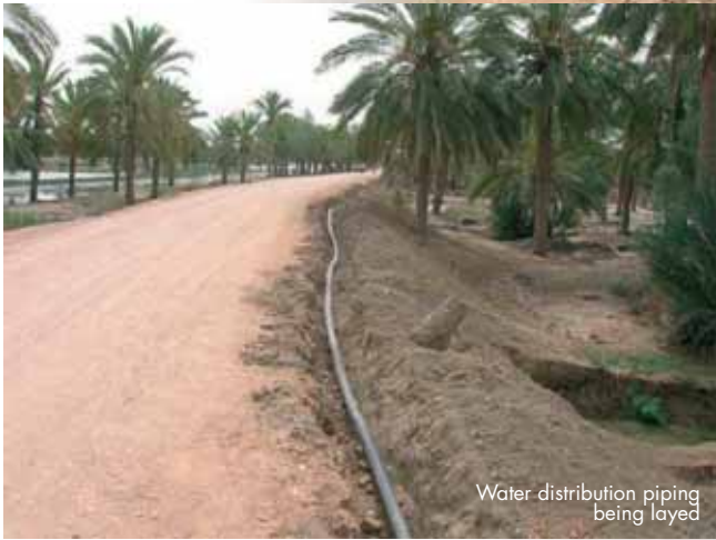
Piping being layed HDPE
