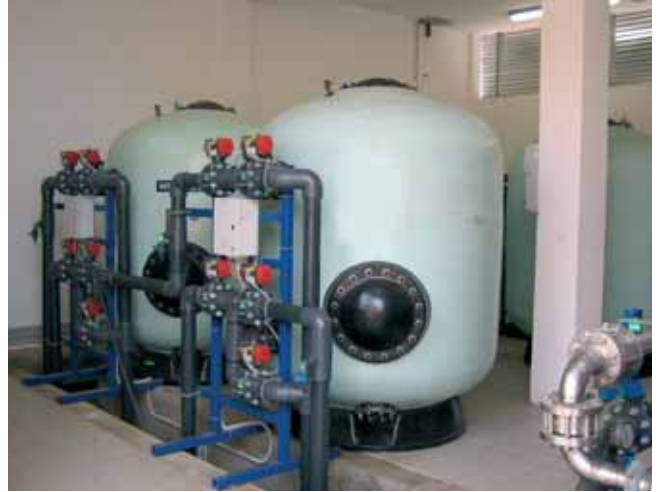
Above: Pretreatment line for sea water. Left: Remineralization and pressurization network. Below: Group of reverse osmosis lines
